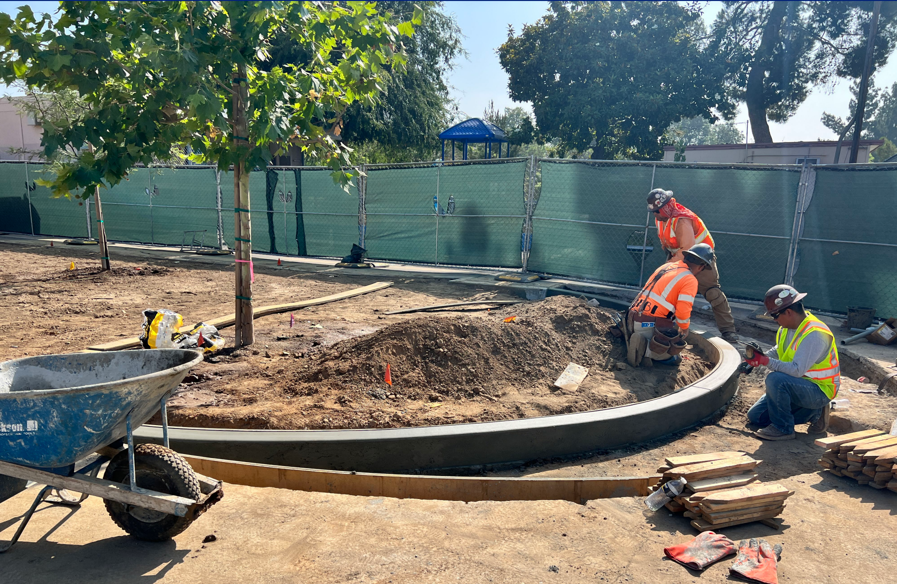
Hamasaki Elementary School landscaping bed is prepared for shrub installation
